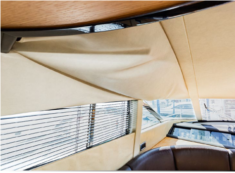
The linings on the bulkheads and ceilings had started to sag
